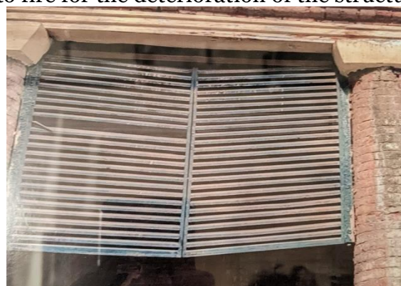
Figure 9. Condition of louver
