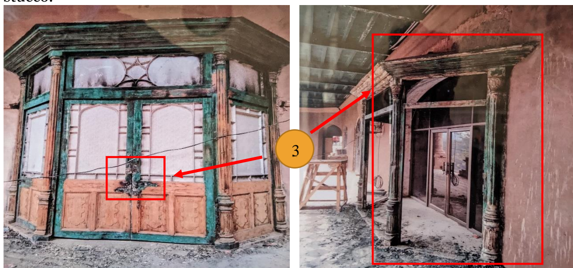
Figure 6. Condition of Portico
