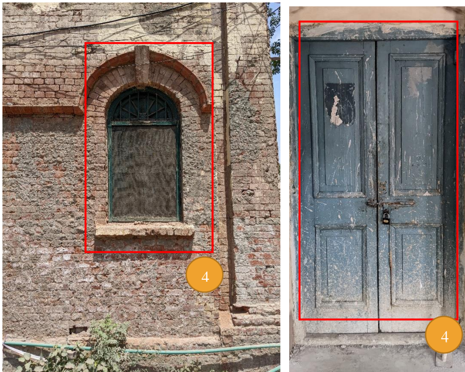
Figure 7. Present Condition of Windows and Doors
